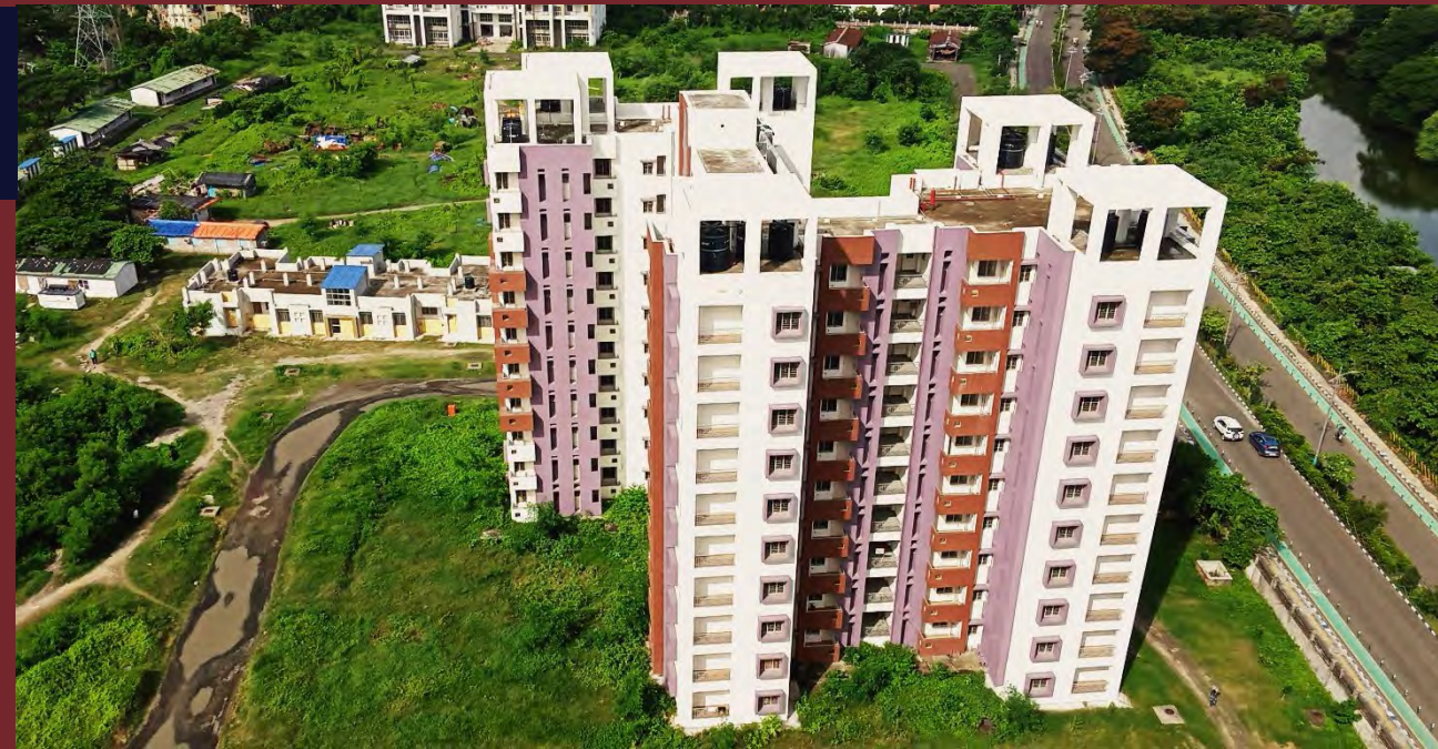
Construction of family quarters Type-II 204 Nos. (G+17), Type-III 30 Nos. & Type-IV 30 Nos. (G+9), Type-V 2 Nos. including internal water supply, sanitary installation, drainage and electrical works for CRPF
