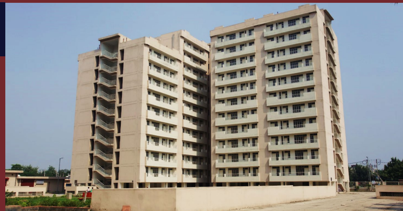
Construction of 483 Multistoried Houses Pkt-1, Sector-A-9, Narela, Delhi
