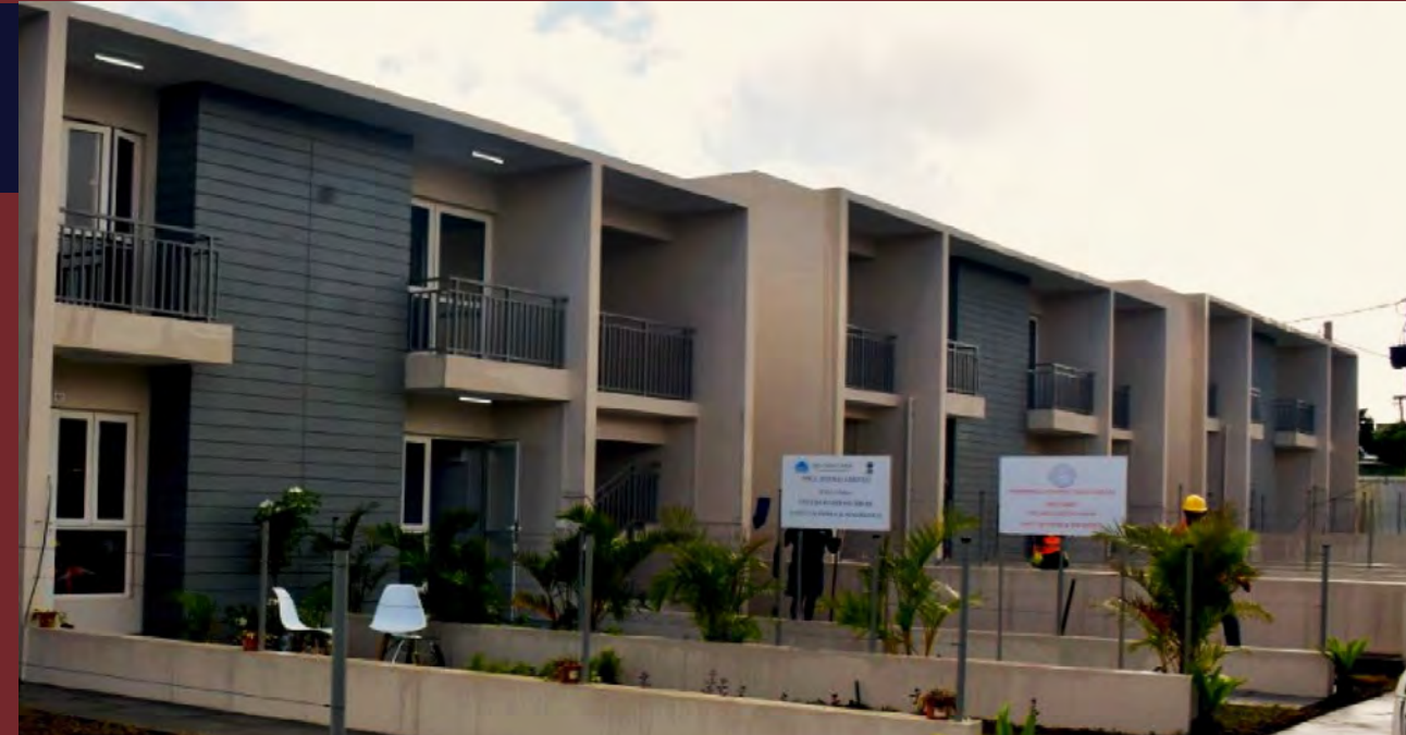
Construction of Social Housing at Mare Tabac and Dagotiere, Mauritius
