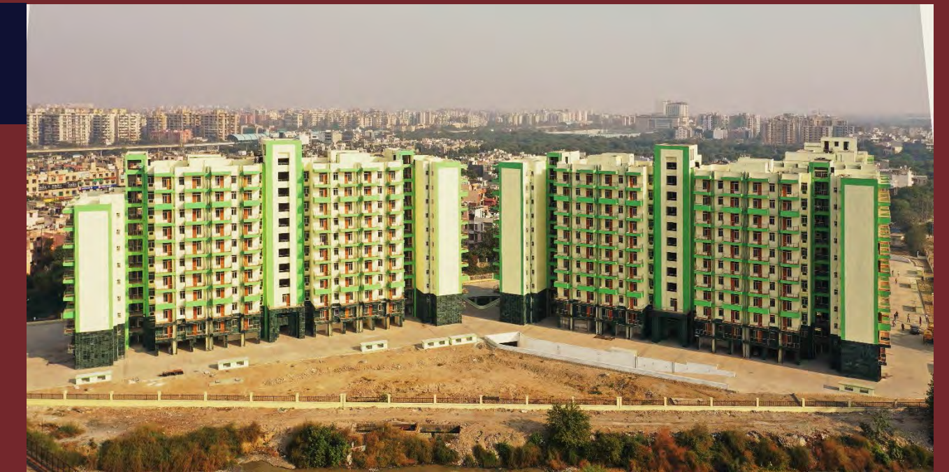
C/o 352 Multistoried two bedroom apartments including internal electrification adjoining pocket-3, sector 19B, Dwarka Phase-II
