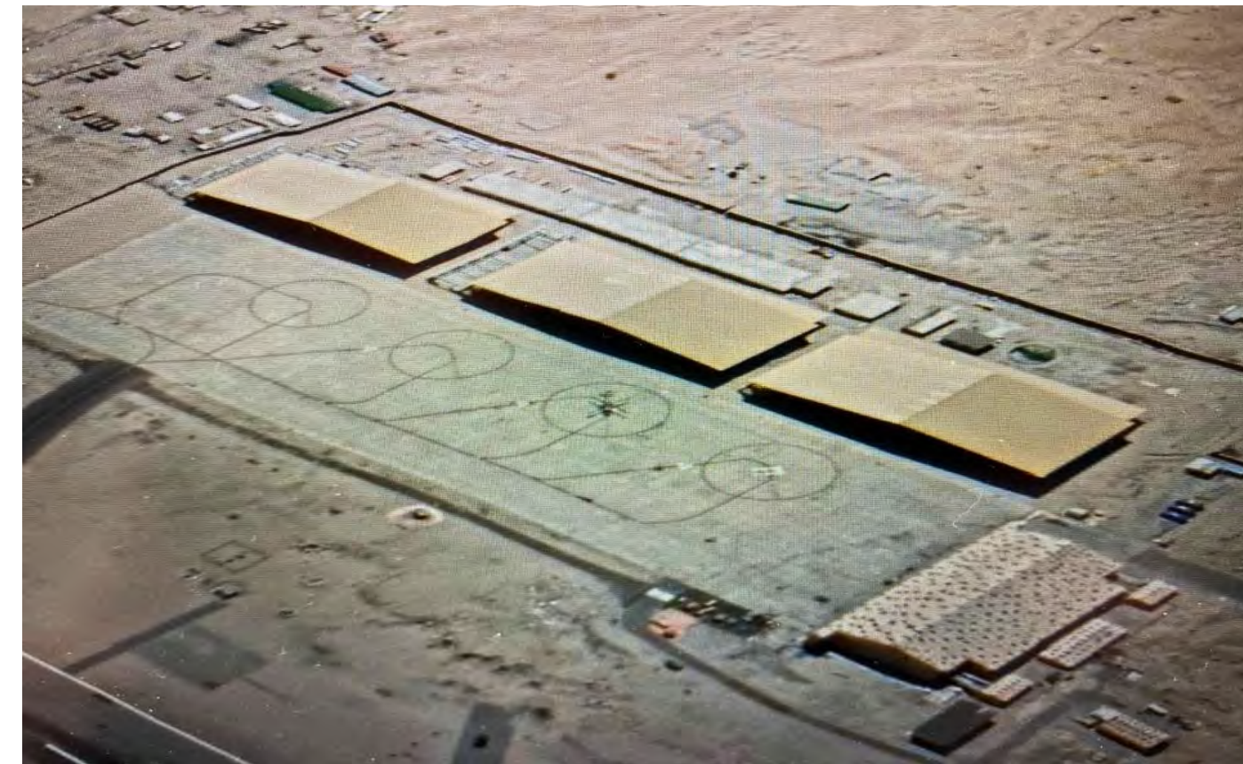
Construction of 3X Twin hangers at AF Station, (Thoise)
