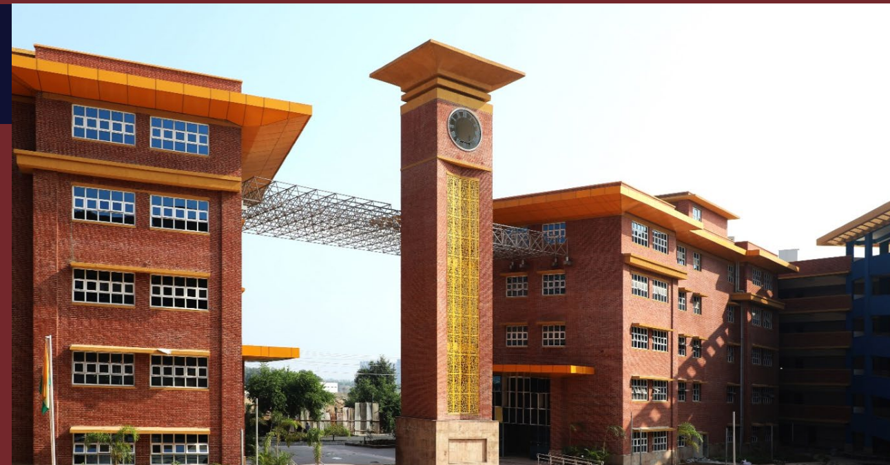
Delhi Public School Building at plot no 224-228, Knowledge Park-V, Greater Noida for DPS Society - Package-I (Civil)
