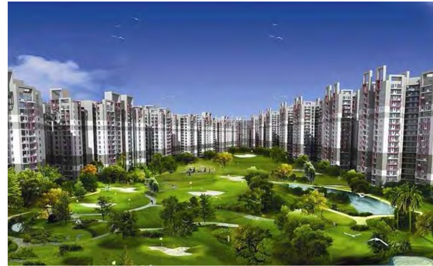
Construction/ Rectification Greater Noida, (UP)
