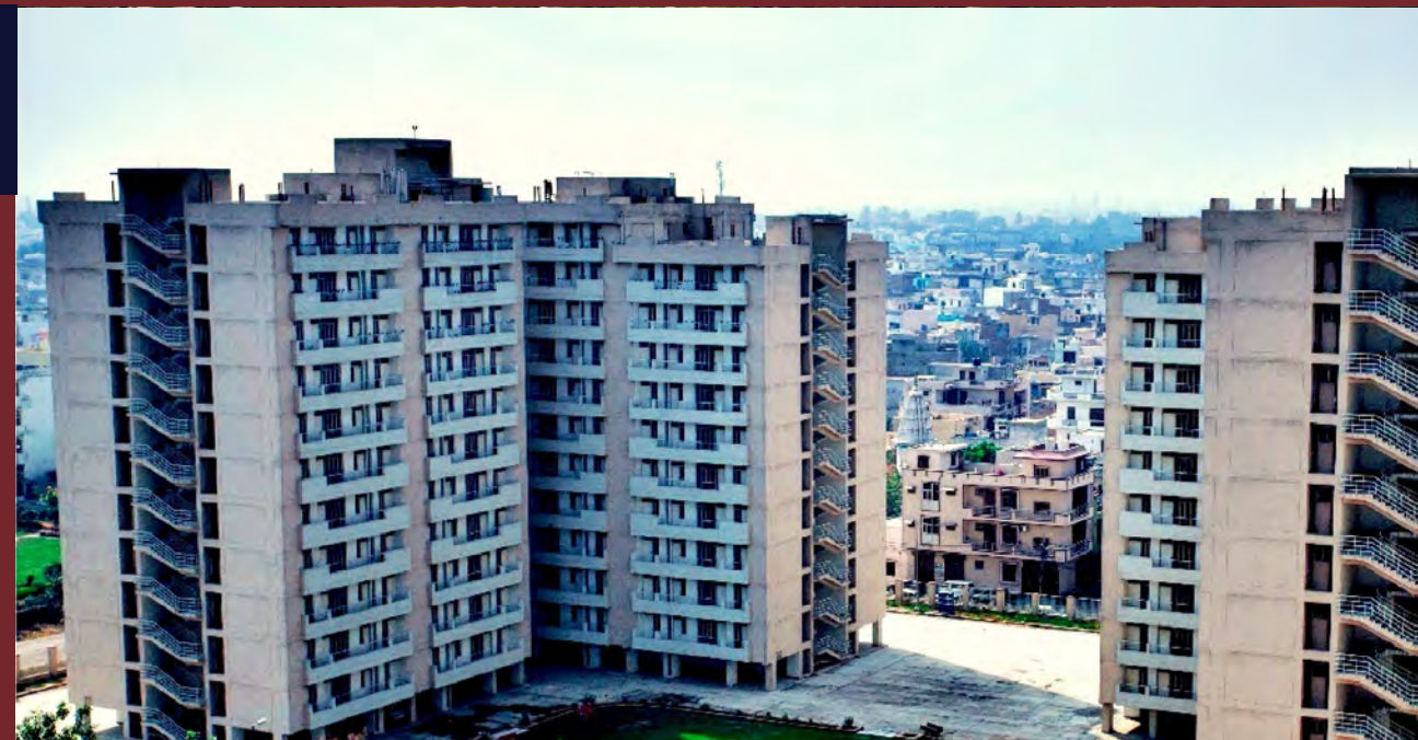
Completion of Balance works for Construction of dwelling Units including allied services for OFFRs, JCOs / ORs at Jodhpur (ARMY)
