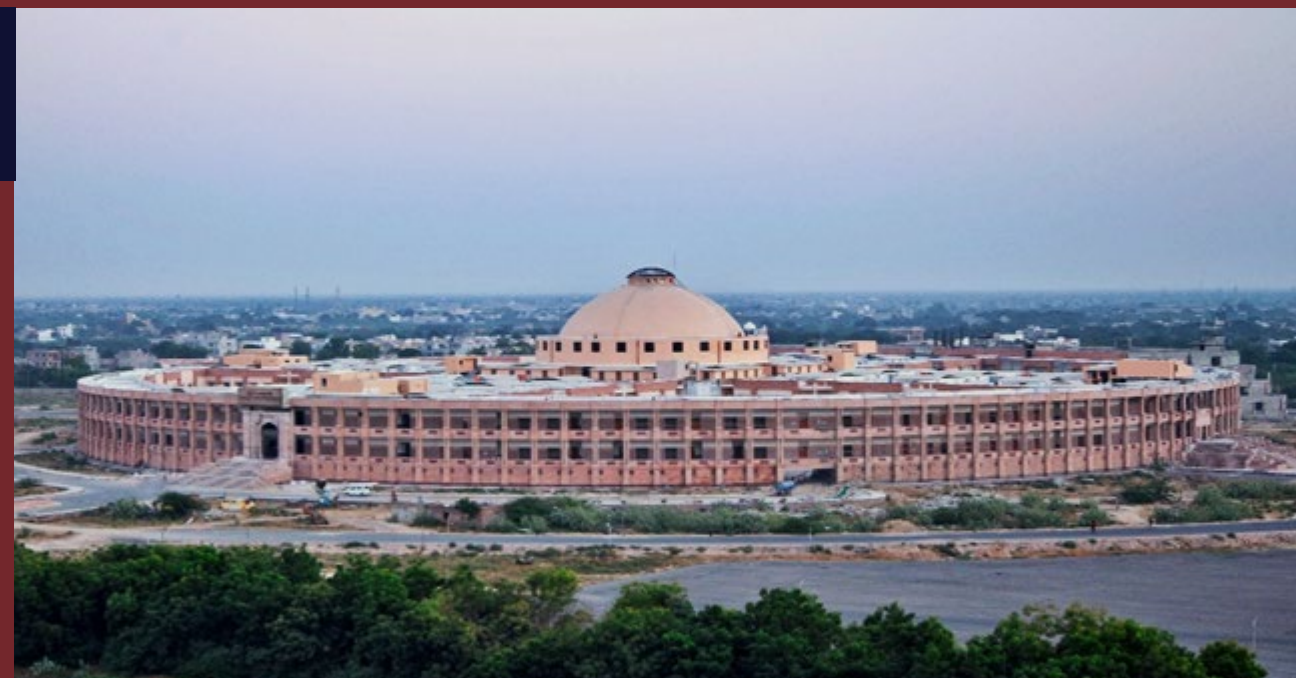
STRUCTURAL WORK FOR CONSTRUCTION OF NEW HIGH COURT BUILDING AT JHALAMAND, JODHPUR
