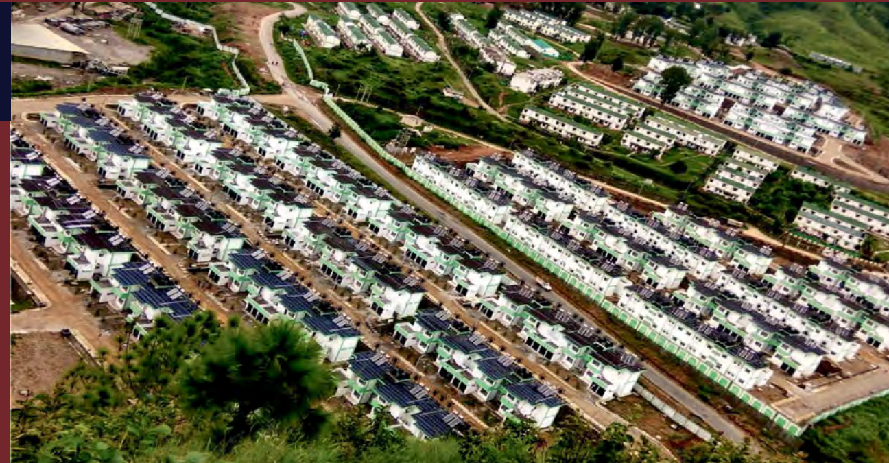
CA No. CEB/PGH/03 of 2013-14: Provn of Md Accn for Officers, JCOs and ORs MAP (Phase-II) at Pithoragarh
