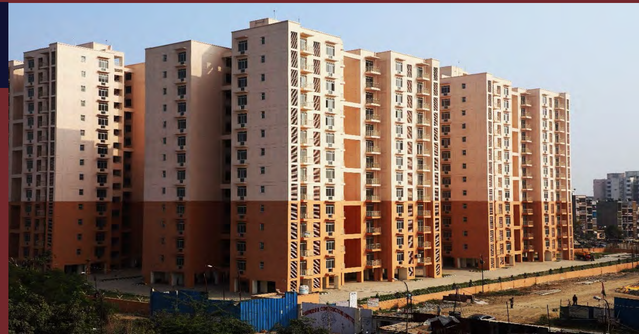
Construction of HIG houses at Pocket 9-B Jasola
