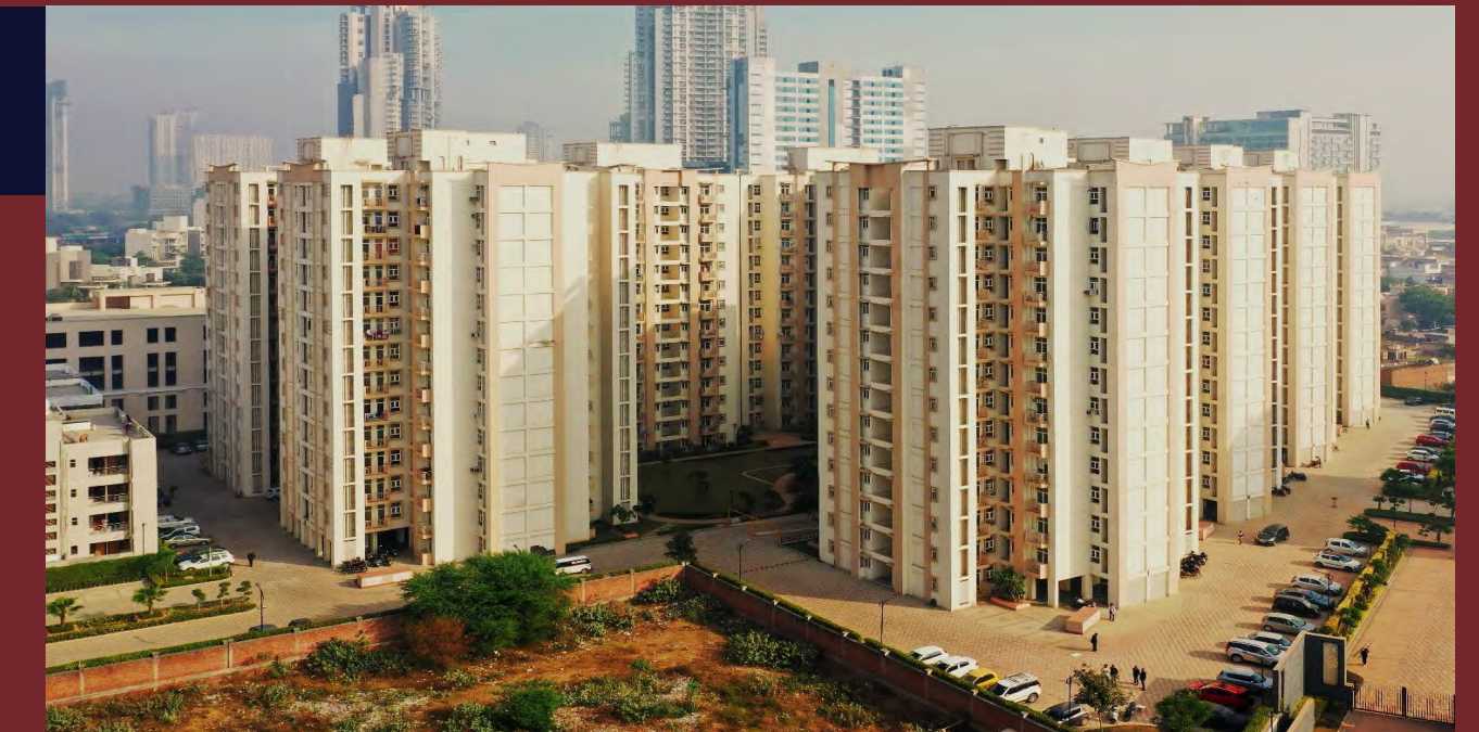
Construction of Shree Vardh1han Mantra; Sector-67, Gurgaon for High Rise Towers (G+14 Storied), Low Rise Towers, EWS Towers & Open Basement
